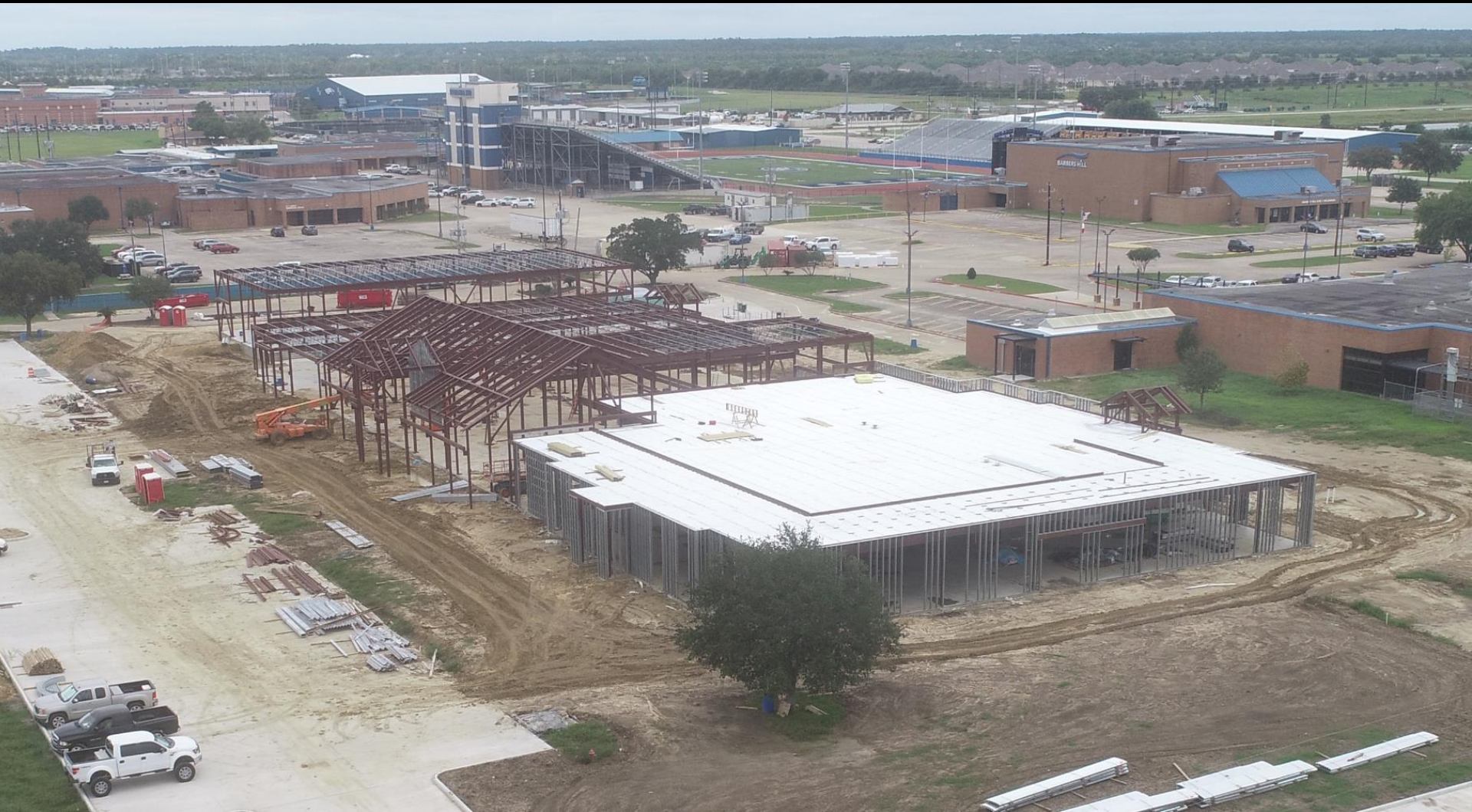
Aerial - Structural Steel Frame and Metal Roof Decking Area C
