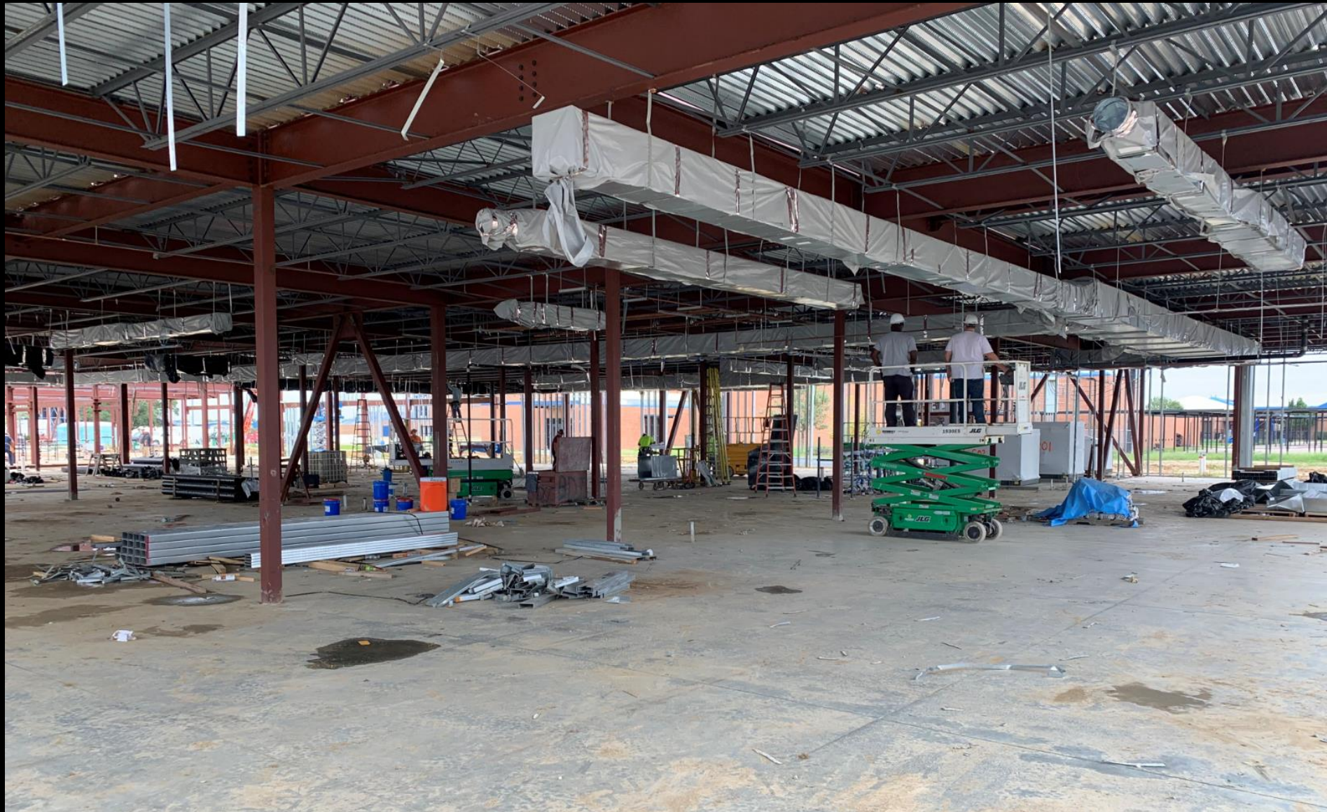
Metal Roof Decking Area C – Duct Work Installation in Progress; Exterior Light Gauge Steel Framing in Progress
