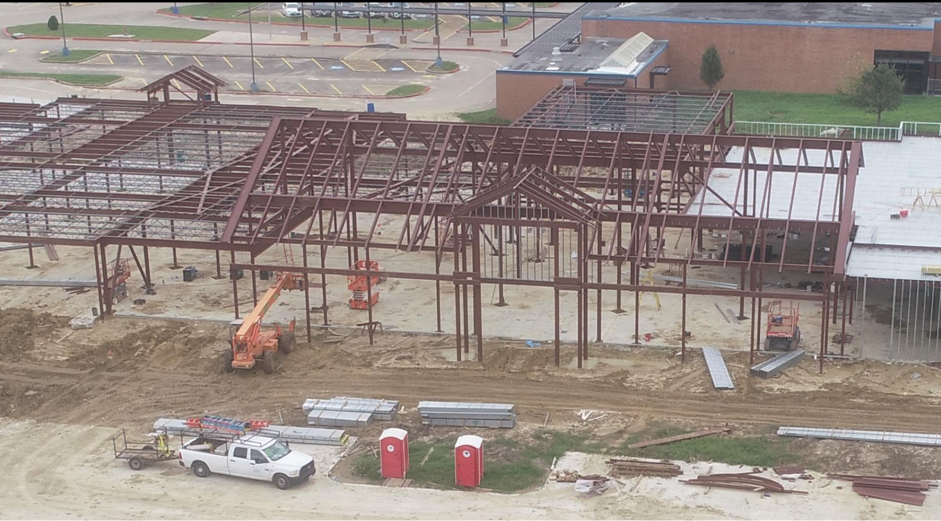
Aerial - Structural Steel Frame – Main Entry
