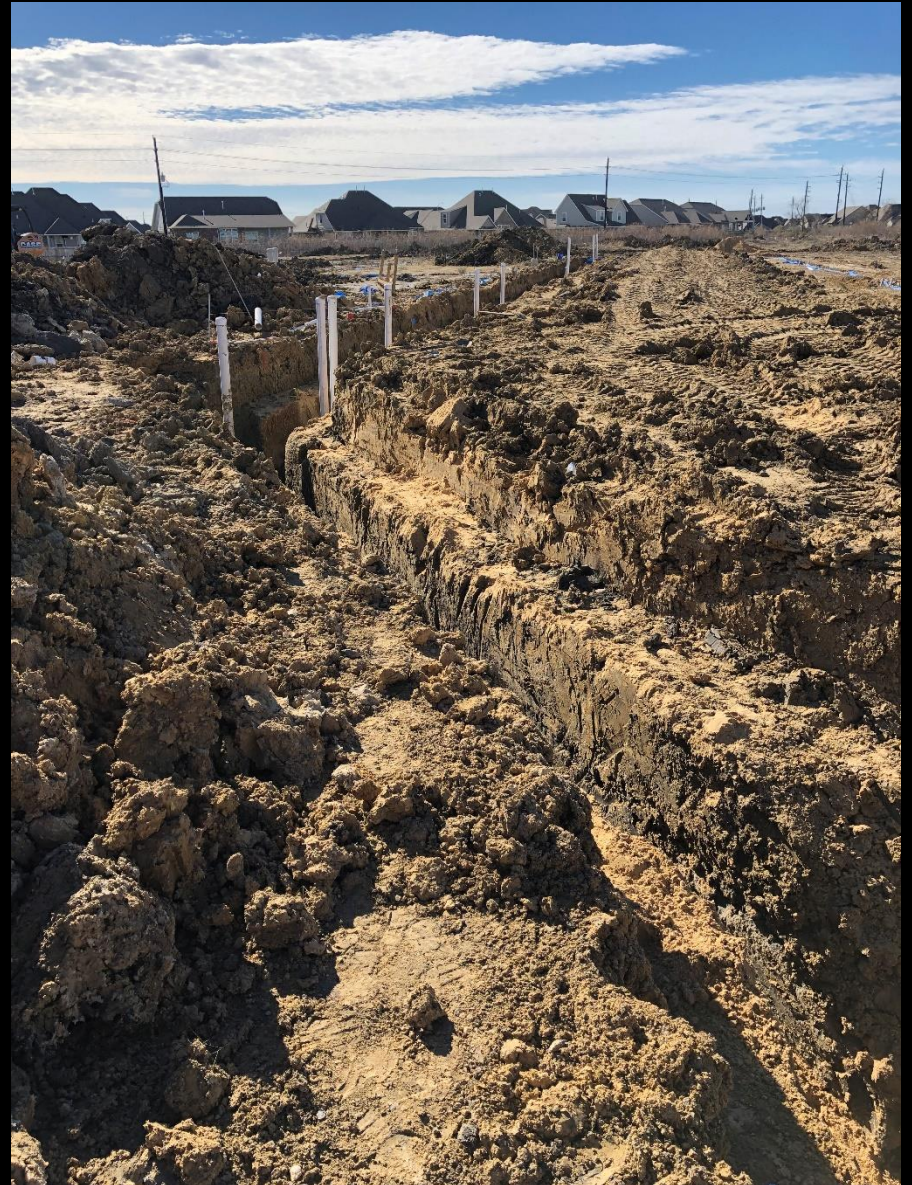
Main Power Service Underground
