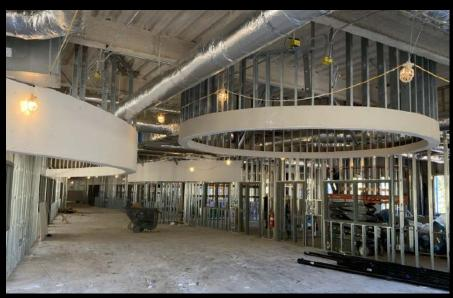
Installation of Main Duct Line, Metal Studs at CMU at Food Service Area, Spray Fire Proofing to Roof Structure, Interior Gyp. Bd. Fur Downs
