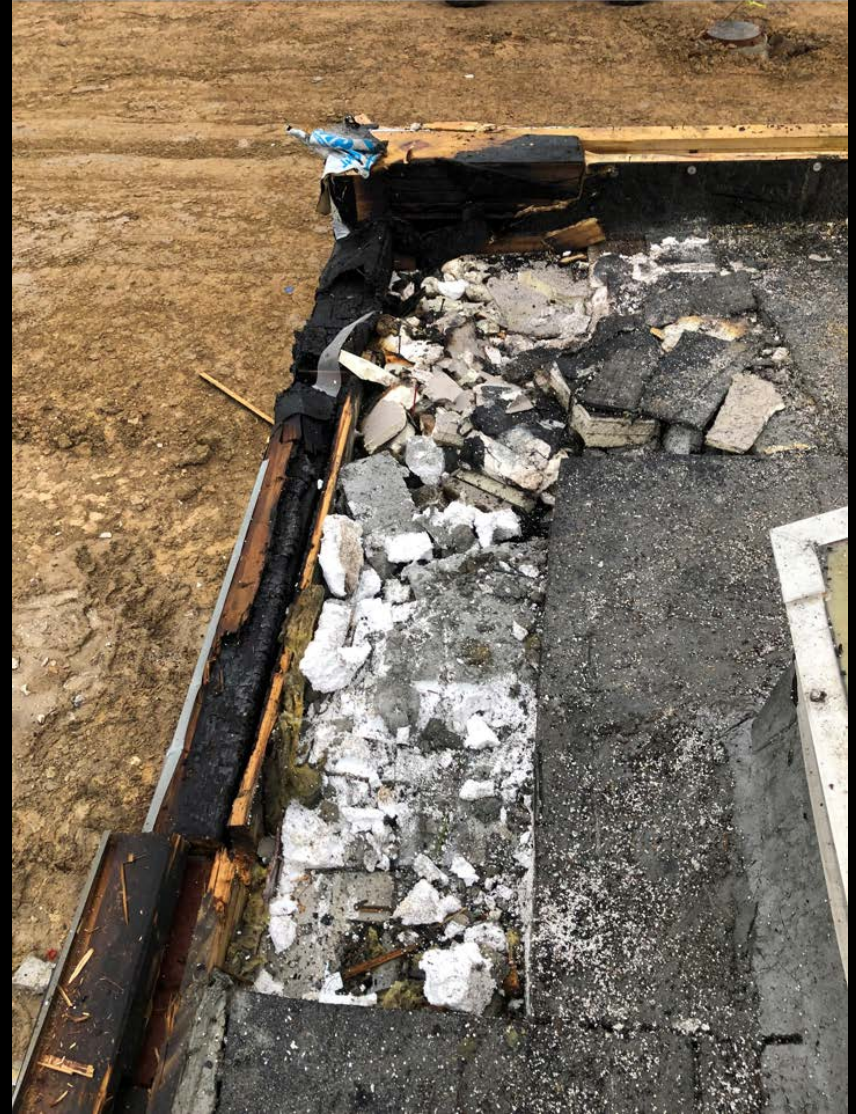
Primary School – Entry Elevation – 5-15-20 Lightning Strike Damage
