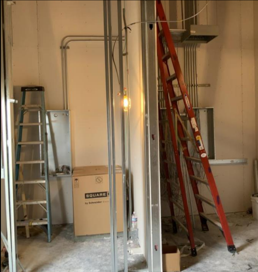
Installed electrical transformer and pulling of wires into electrical panels:
