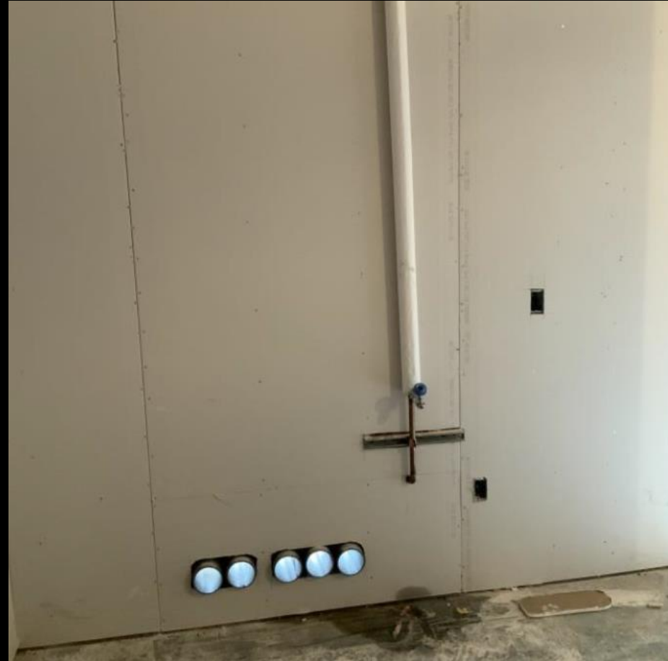
Interior and exterior hose bib installed in mechanical room:
